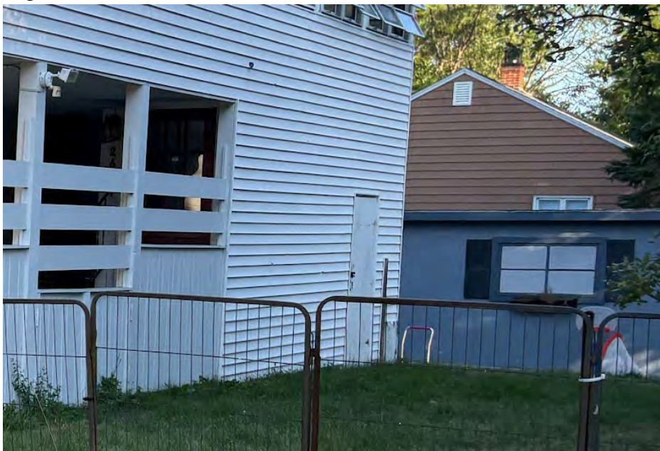
View of storage space only accessible from 276 Dennett St
